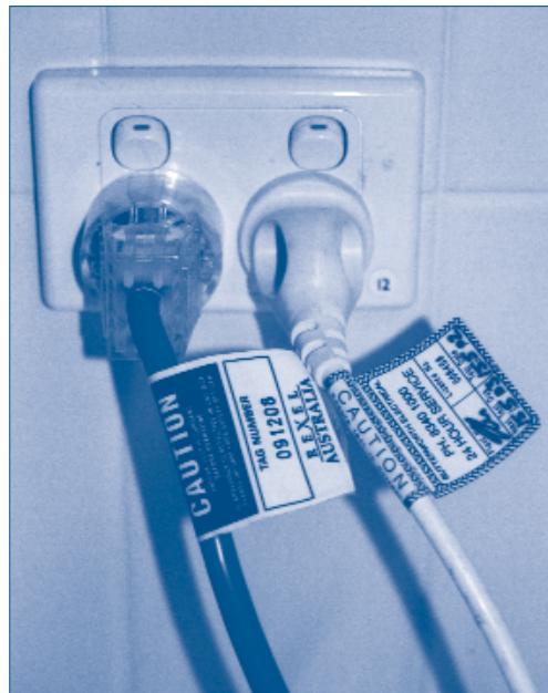
Examples of suitably tagged electrical leads
